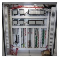
A new electrical room was constructed for the new Motor Control Center (MCC), PLC panel, network switch cabinet, and associated electrical equipment. A new dedicated HVAC system was installed for the electrical room in order to protect the electrical equipment from the environmental impacts and extend the life of the equipment. A new PLC panel was installed along with all new instrumentation and field controls. All electrical and I&C components in the building were replaced.
